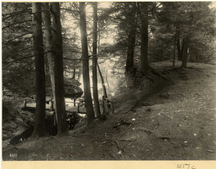
Figure 9. Photograph of Hemlock Gorge, wooden bridge. Courtesy of National Park Service, Frederick Law Olmsted National Historic Site
