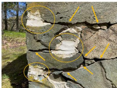
Photo 15: Severely eroded mortar (arrows) and non-matching replacement mortar (circled)
