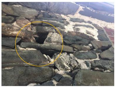
Photo 16: Missing chinking in exterior stone masonry
