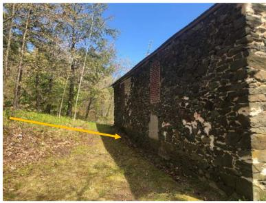
Photo 26: Exterior grade slopes toward the west wall of the building (arrow), where water seepage is occurring through the natural ledge outcropping at the interior
