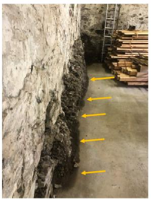
Photo 4: Moisture on floor at natural ledge outcropping along west wall
