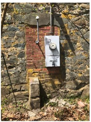
Photo 21: Electrical equipment and conduits attached to, penetrating through, and marring the historic appearance of the exterior masonry walls
