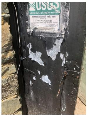
Photo 24: Peeling paint on galvanized steel entrance door
