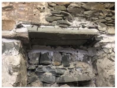
Photo 7: Lintel replaced with stone
