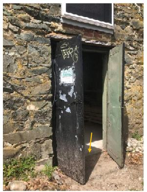
Photo 2: Entry door with vertical offset from exterior to interior (arrow)
