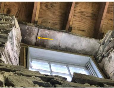
**Photo 6: Cracked stone lintel**
