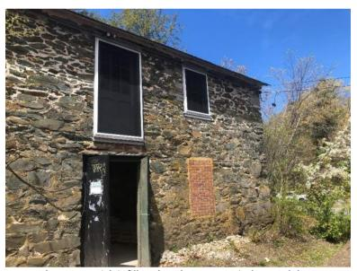
Photo 23: Brick infill and replacement window and door
