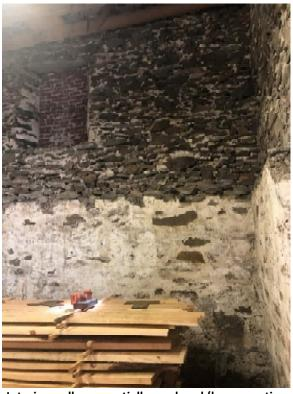
Photo 28: Interior walls are partially rendered (lower portion of photo)
