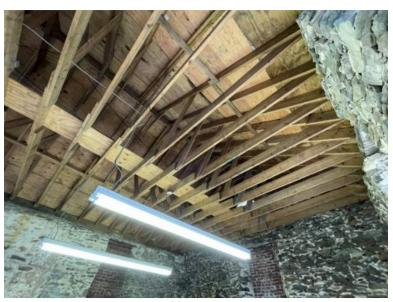
Photo 13: Roof framing and sheathing
