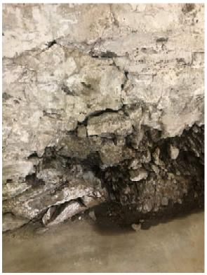
Photo 5: Loose rubble stone masonry above puddingstone ledge
