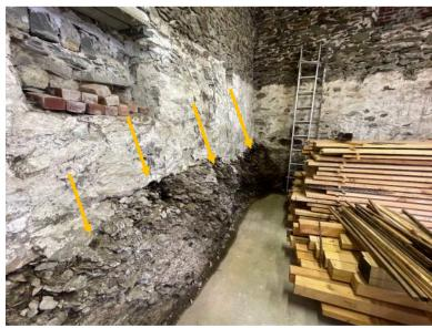
Photo 3: Roxbury puddingstone ledge outcropping at west elevation
