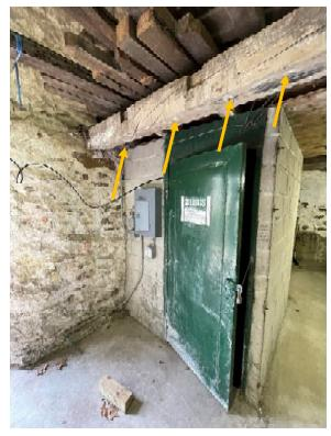
Photo 10: Checked second-floor wood framing
