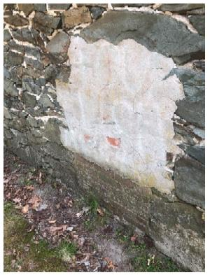
Photo 19: Parge coat at west elevation
