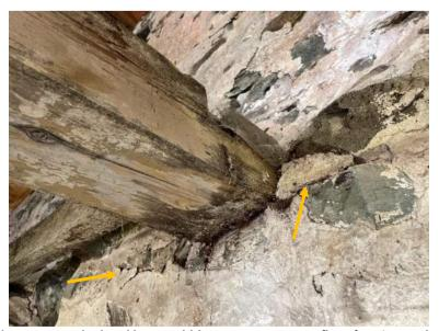
Photo 11: Cracked and loose rubble stone masonry at floor framing pocket
